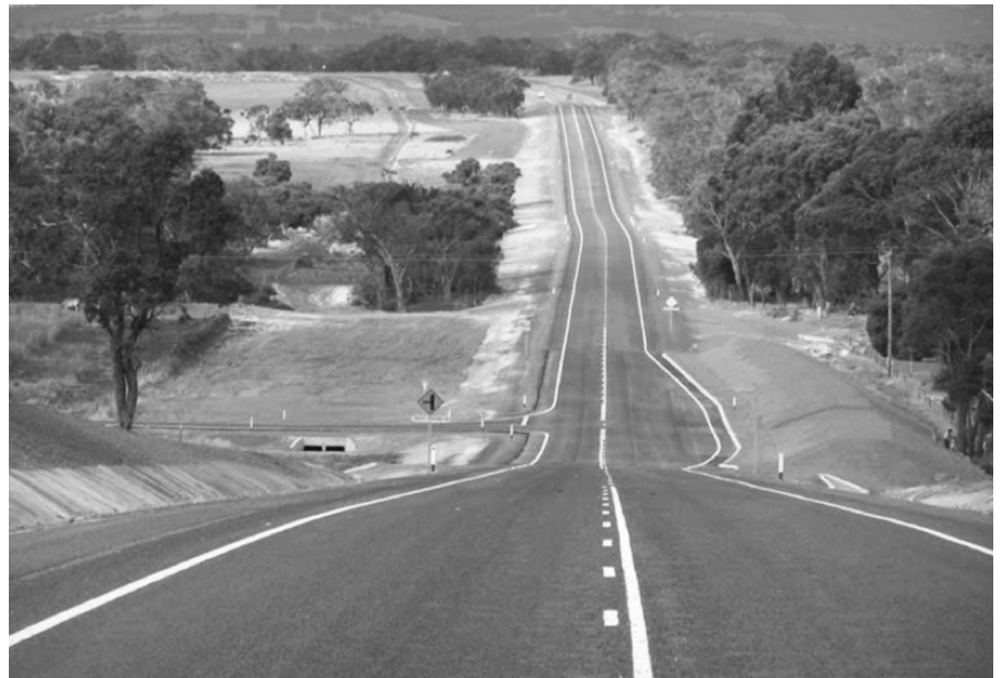
Stage 1: Constructed in 2007
